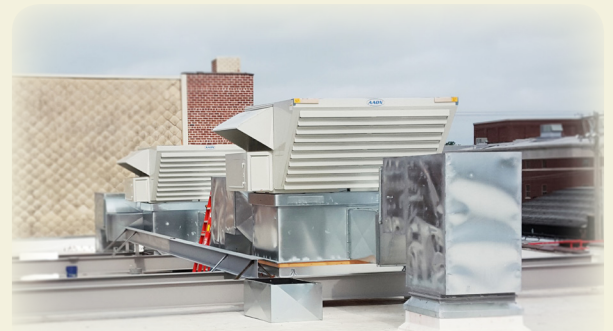
Above: Completed HVAC units
