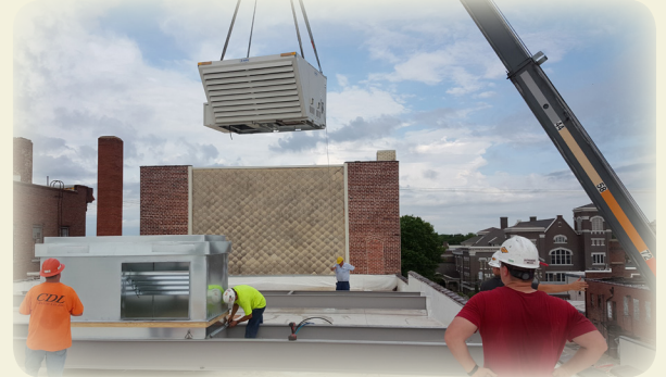
Above: Lowering of the HVAC unit onto the roof
